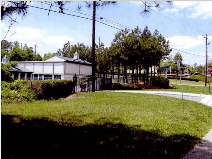
View of Storage Facility
