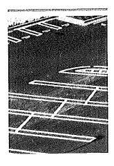
These changes have had a profound impact on parking dimensions. In the past, full-size parking stalls in some locations were 9 to 10 feet wide and 18 to 20 feet long. With smaller automobiles, an average width of 8.5 feet and a length of 16 to 17 feet is more appropriate for general use, with even smaller dimensions acceptable in
