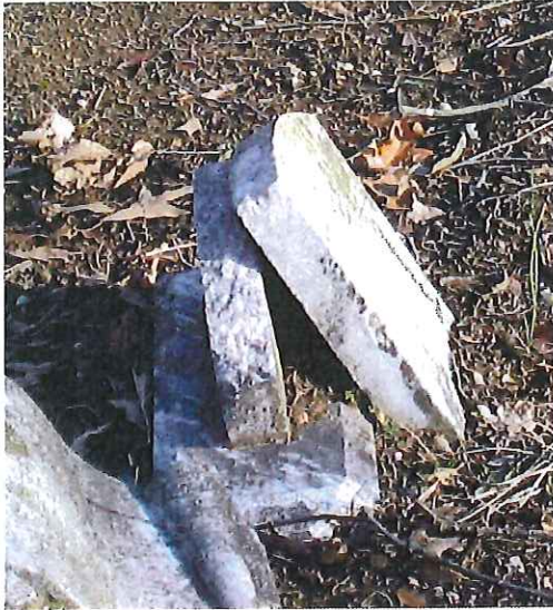
Figure 4.2 This die in socket monument found in the northern portion of Methodist Cemetery has been broken by vandals. Until it can be repaired it should either be stored off site, or buried next to its base.
