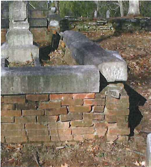
Figure 4.13 The coping surrounding this family plot near the original site of the Mt. Carmel Baptist Church is in need of repointing.
