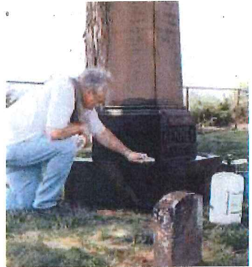
Figure 4.6 As in this example, monuments should be pre-wetted prior to the start of the cleaning process and should be cleaned from the bottom up. Photo courtesy of Connecticut Gravestone Network.
