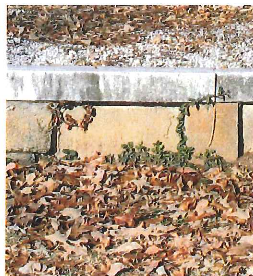
Figure 3.13 Detail of ivy growing into cracks among the concrete masonry unit blocks of the coping of the Gray family plot.
