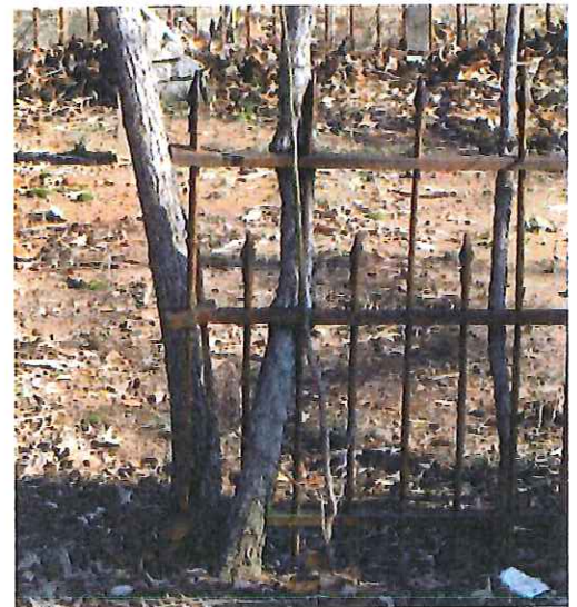
Figure 3.16 Scrub trees have grown up through and around the cast iron fence of the Hook family plot.
