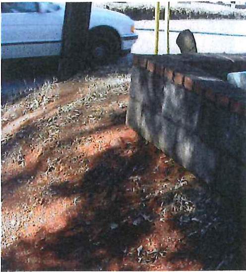
Figure 4.9 This coping is being undermined by erosion along this access road off of Woodstock Street. It is important to halt such erosion.
