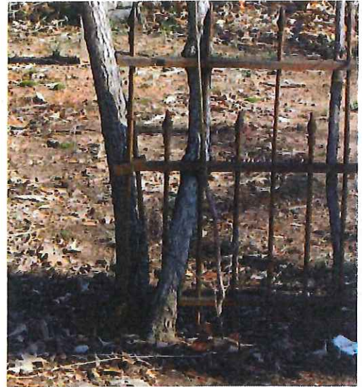
Figure 4.11 These trees should have been removed when they were saplings. If they had been removed the damage to the cast iron fence would not have occurred. Historic cast iron fences are a character-defining feature of any cemetery and should be maintained appropriately.
