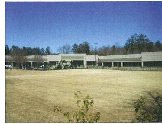
3 VIEW TOWARD MAIN ENTRY
