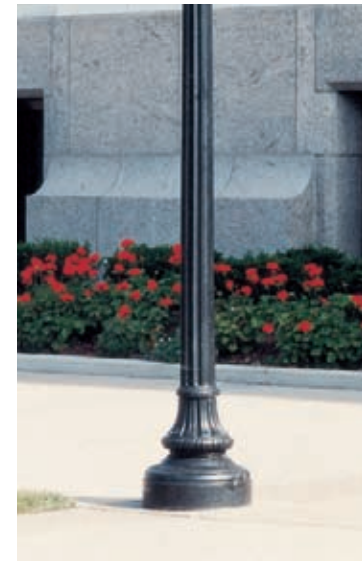
Figure 4-4: Pedestrian light pole base
