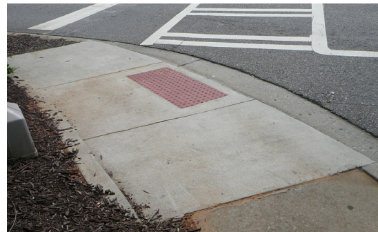
Figure 7-3: Curb ramp detectible warning tile
