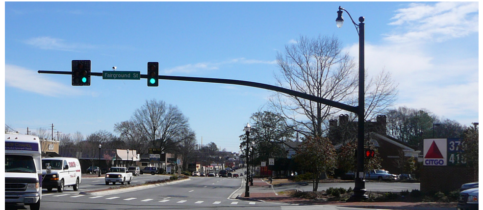
Figure 8-1: Mast arm signal pole
