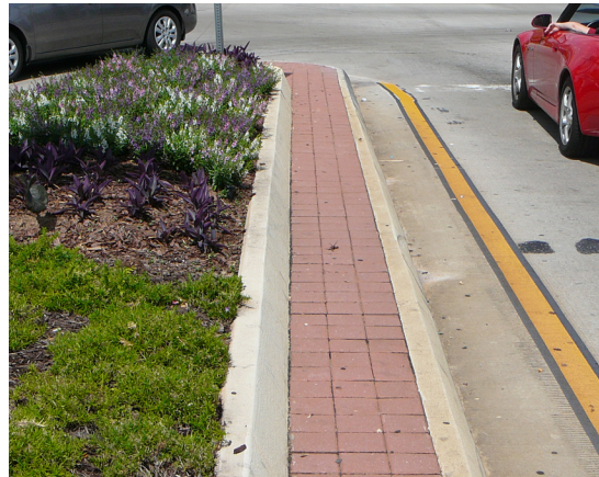
Figure 3-6: Double concrete curb median
