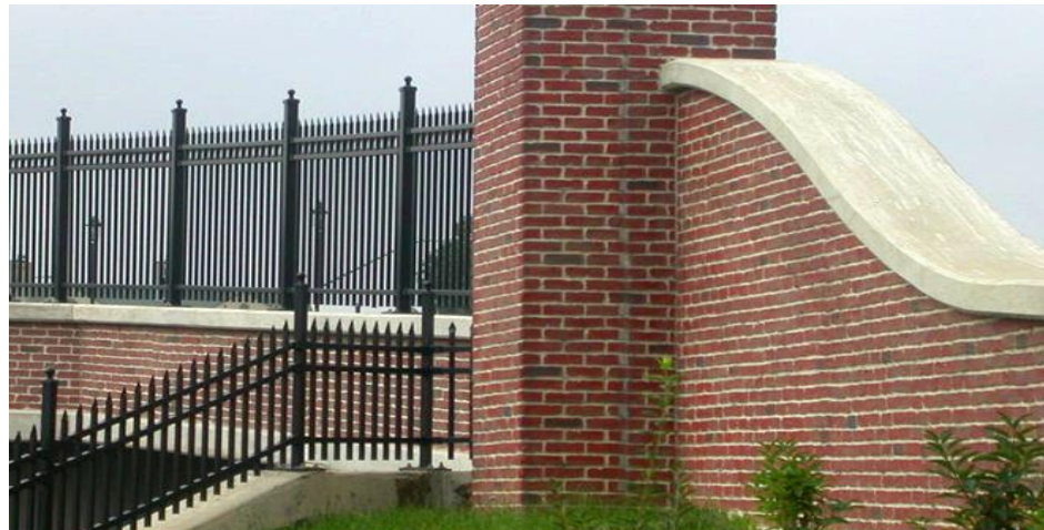
Figure 11-4: Example of thin brick form liner parapet wall character
