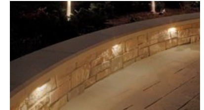
Figure 10-2: Recessed lighting along walls
