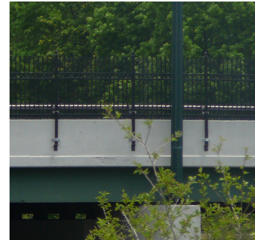
Figure 11-2: Application of short-term bridge fence mounted to bridge parapet wall
