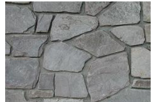
Figure 10-5: Stone retaining wall character
