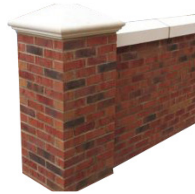
Figure 10-1: Brick/Precast Concrete Guard Wall, Coping, and Pier
