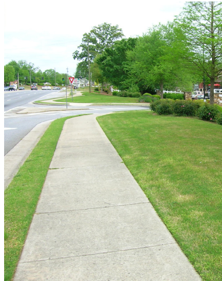
Figure 3-2: Concrete sidewalk character in Overall Corridor
