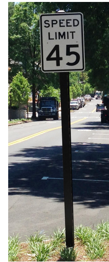
Figure 9-2: 2-Inch aluminum square post
