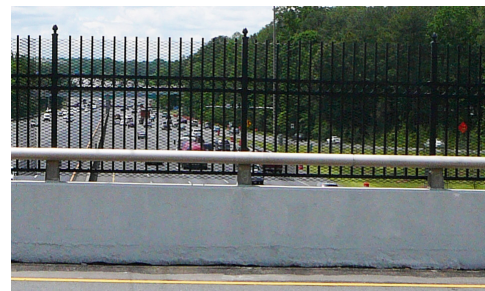
Figure 11-1: Short-term bridge fence character. Enlargement above.
