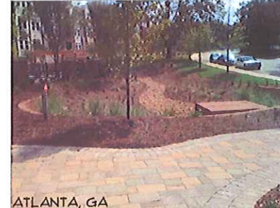
ATLANTA, GA BIORETENTION SWALE
