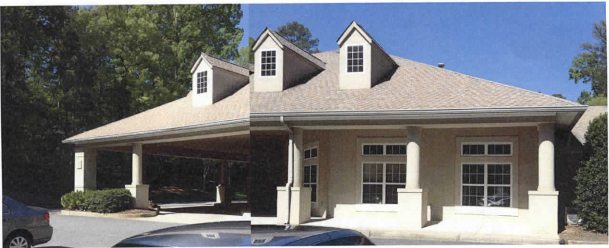
EXISTING TAPESTRY HOUSE – MAIN ENTRANCE
