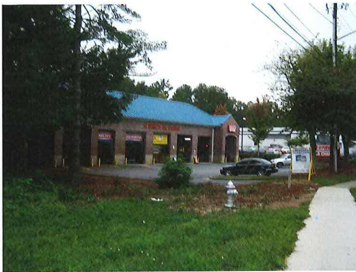
View of property to the west
