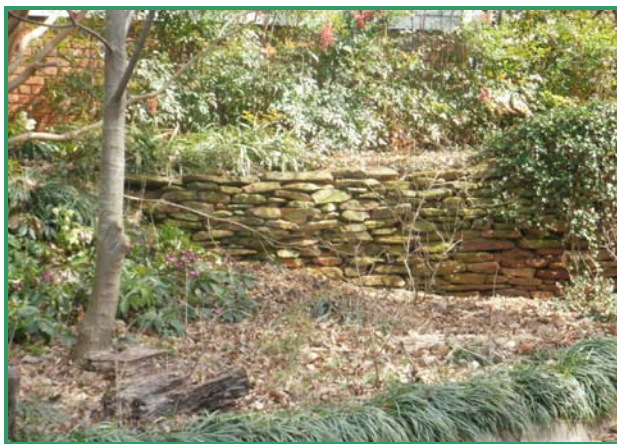
These walls appear to be stacked stone and have strong horizontal lines.
